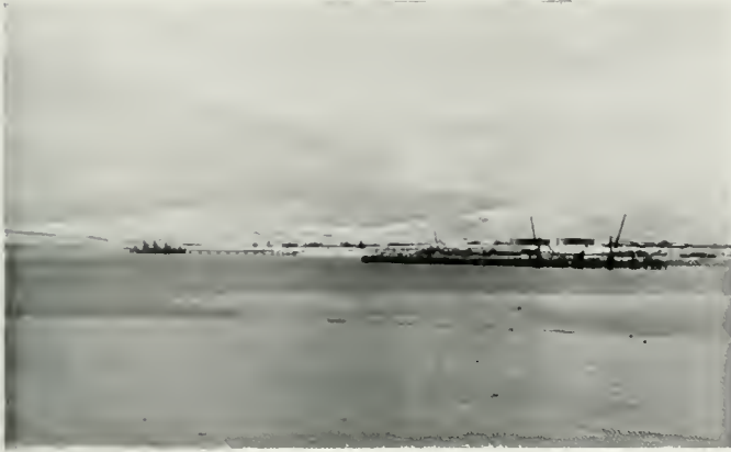
THE NEW STONE WALL AND PIER, LYNESS.
